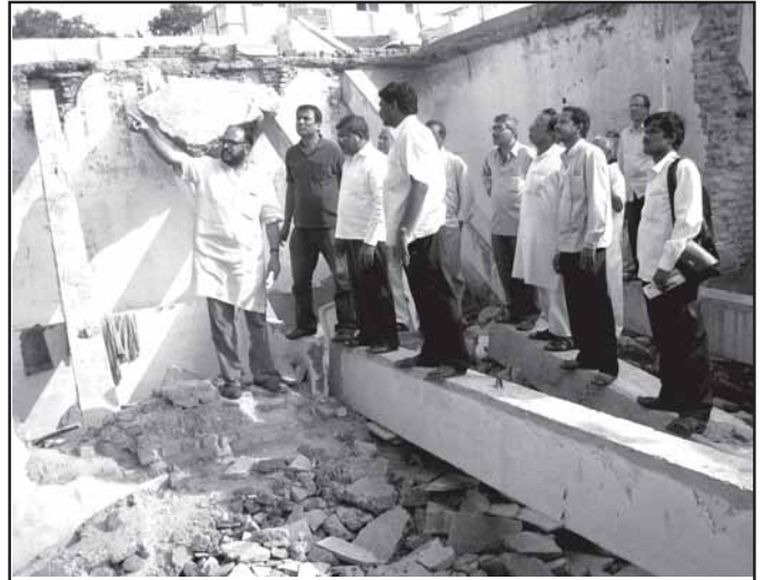
The collapsed portion inside Old Jailkhana
