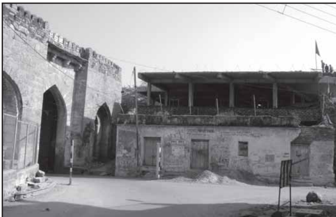
The nursing home under construction at Fateh Darwaja
