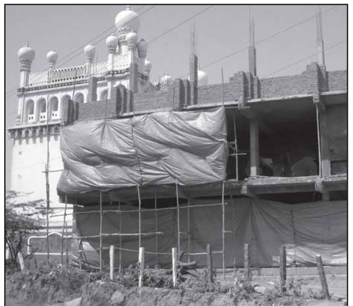
Construction of shopping complex near Jamia Masjid
